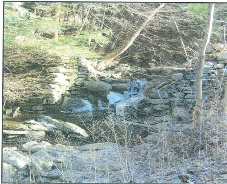
Remnant dam on Heffers Brook along Route 128, North Cornwall.
