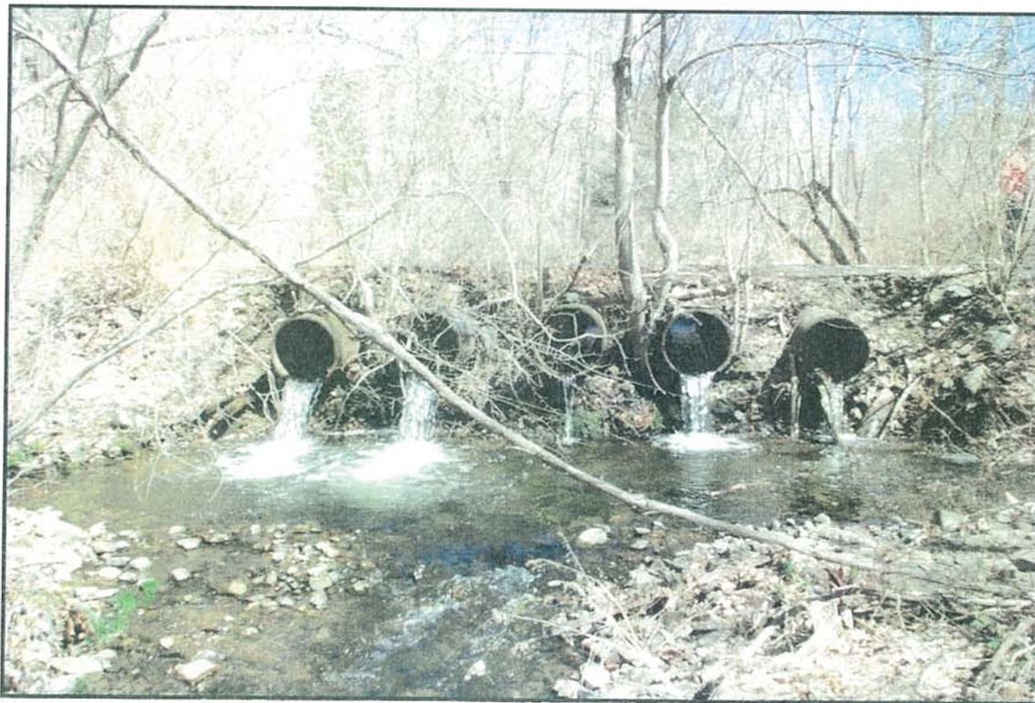
An example of the impact of culverts: habitat loss and a fish migration barrier.
